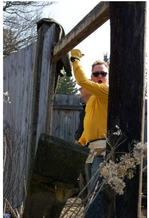
Kevin S taking down the fence boards
